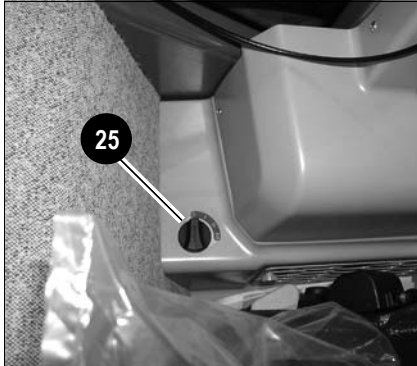
Fig. 69: Air conditioning rotary switch
