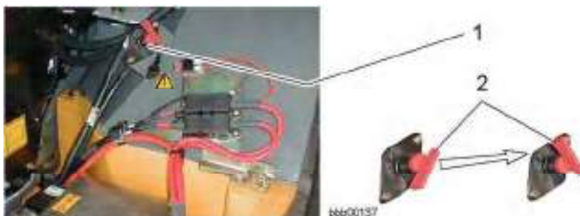
Battery main switch
