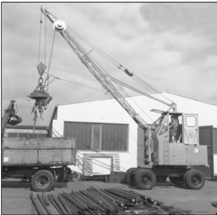
1962: rope-driven S833 with elevated operator cab
