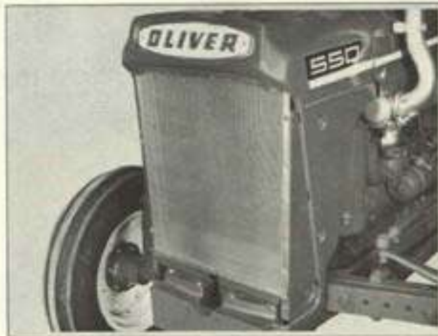
Figure 5-4 Radiator Screen
