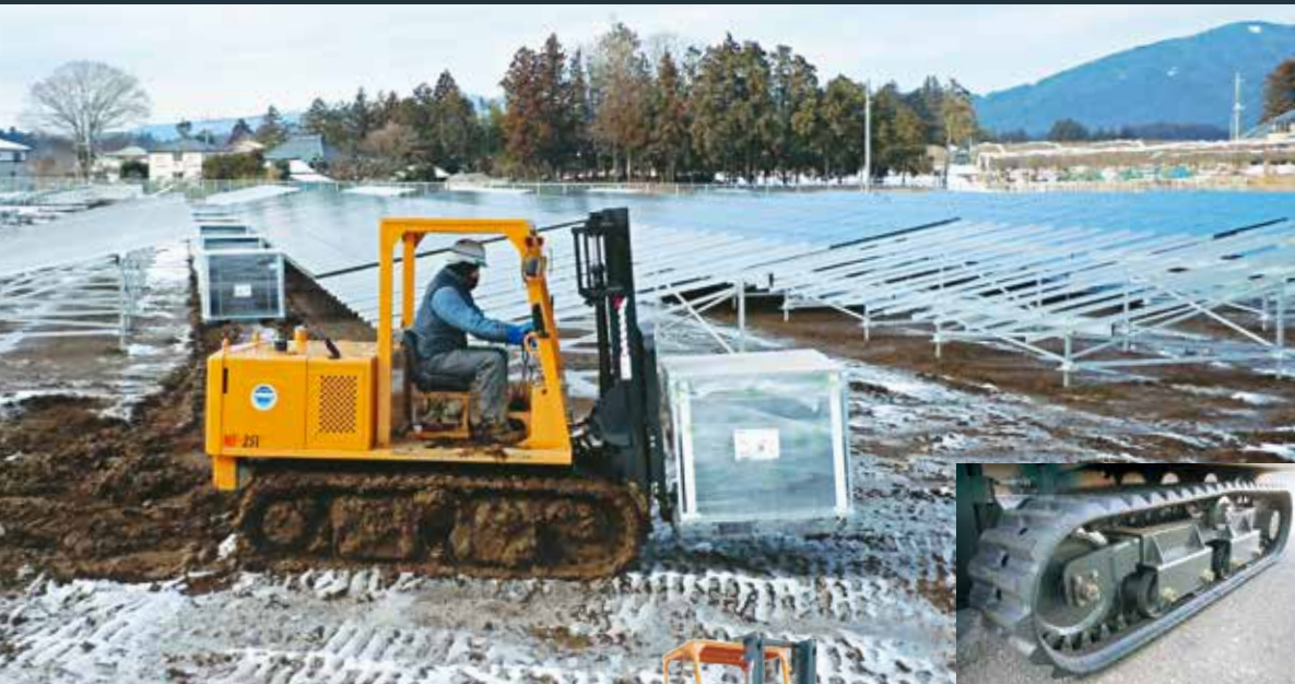
Lifting laying iron plate
