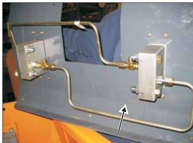
Fig. 6-9 Location of electrical connector to disconnect. Other control handle is similar
