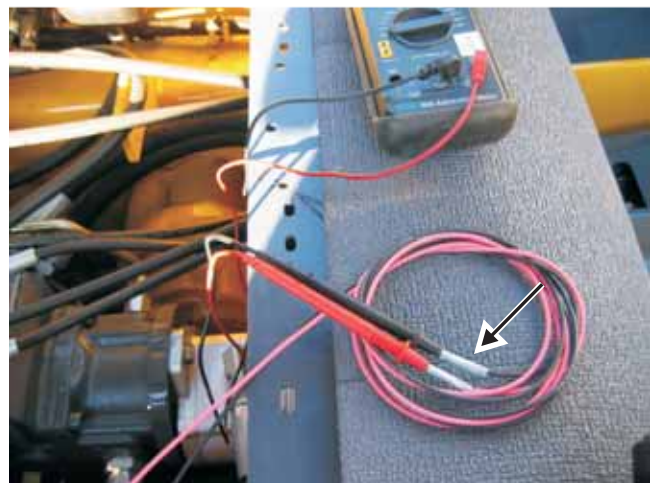
Fig. 9-27 View of the jumper wires attached at the voltmeter pins
