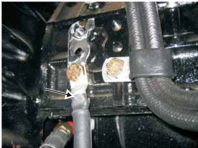
Fig. 10-37 View of the engine ground cable attached to the engine
