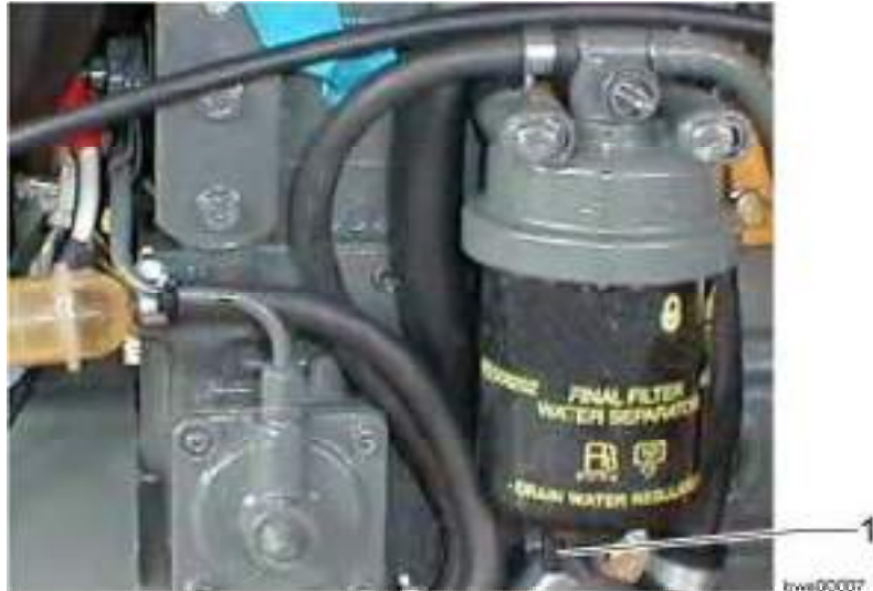
Draining off condensate
