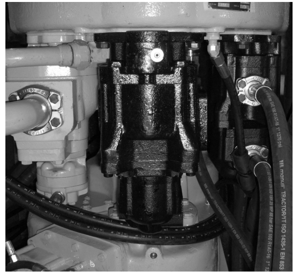
Fig. 7C.62. Installing Equipment Pump
