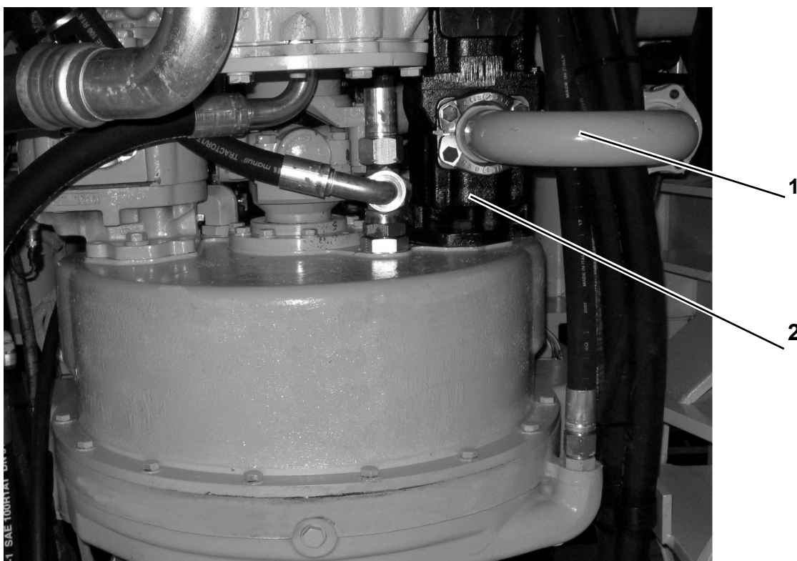
Fig. 7C.78. View from under Machine on Charge and Cooler Pump
