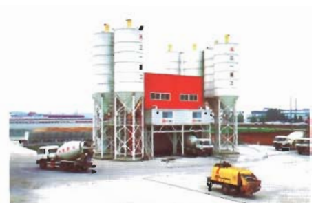
□ In Suizhou Tiancheng Concrete Co.,Ltd., Hubei, China
