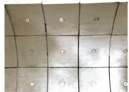
4 Liner Plate inside Mixing Chamber
