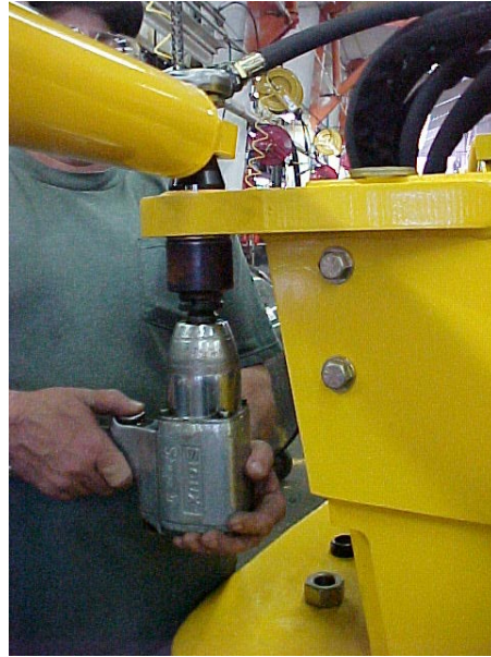
TIGHTENING REAR BOLT.
