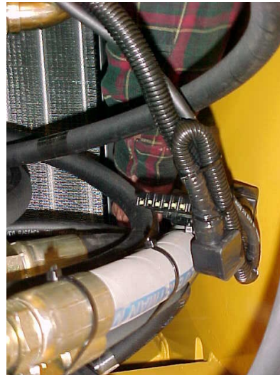
INSTALLING LEFT RADIATOR MOUNT
