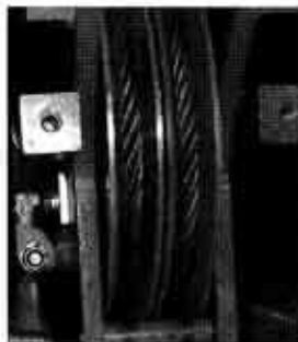
EXTENSION CABLE INSTALLED ON SHEAVE
