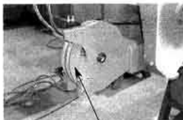
Install Cable Before Sheave Components
