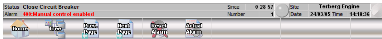
Close Circuit Breaker.bmp
